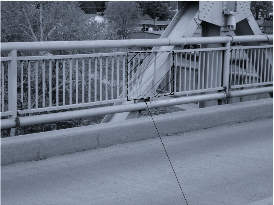
Replace Deteriorated Rail Elements
