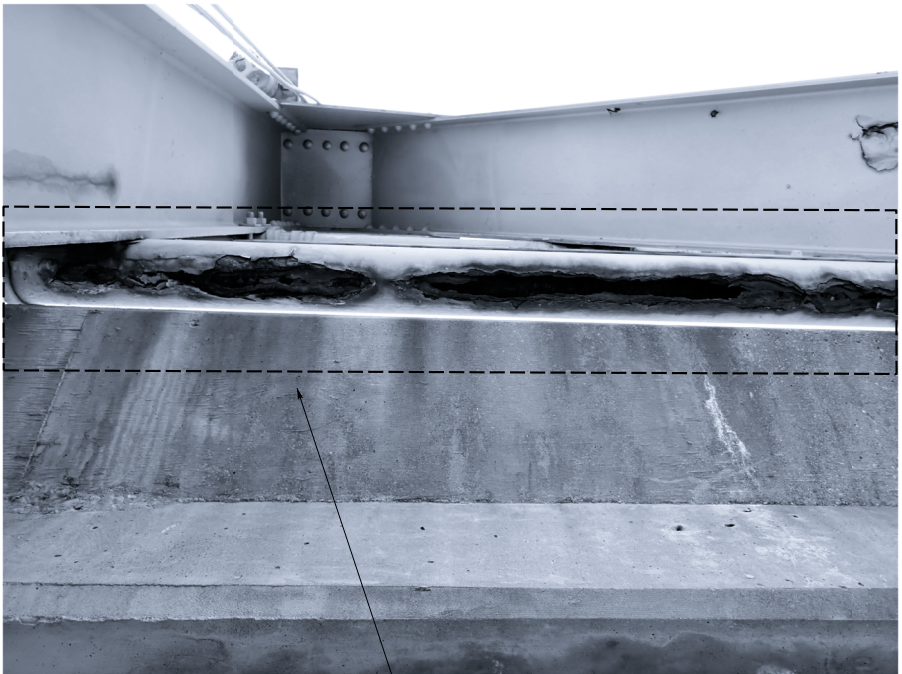
Replace Deteriorated Rail Elements
