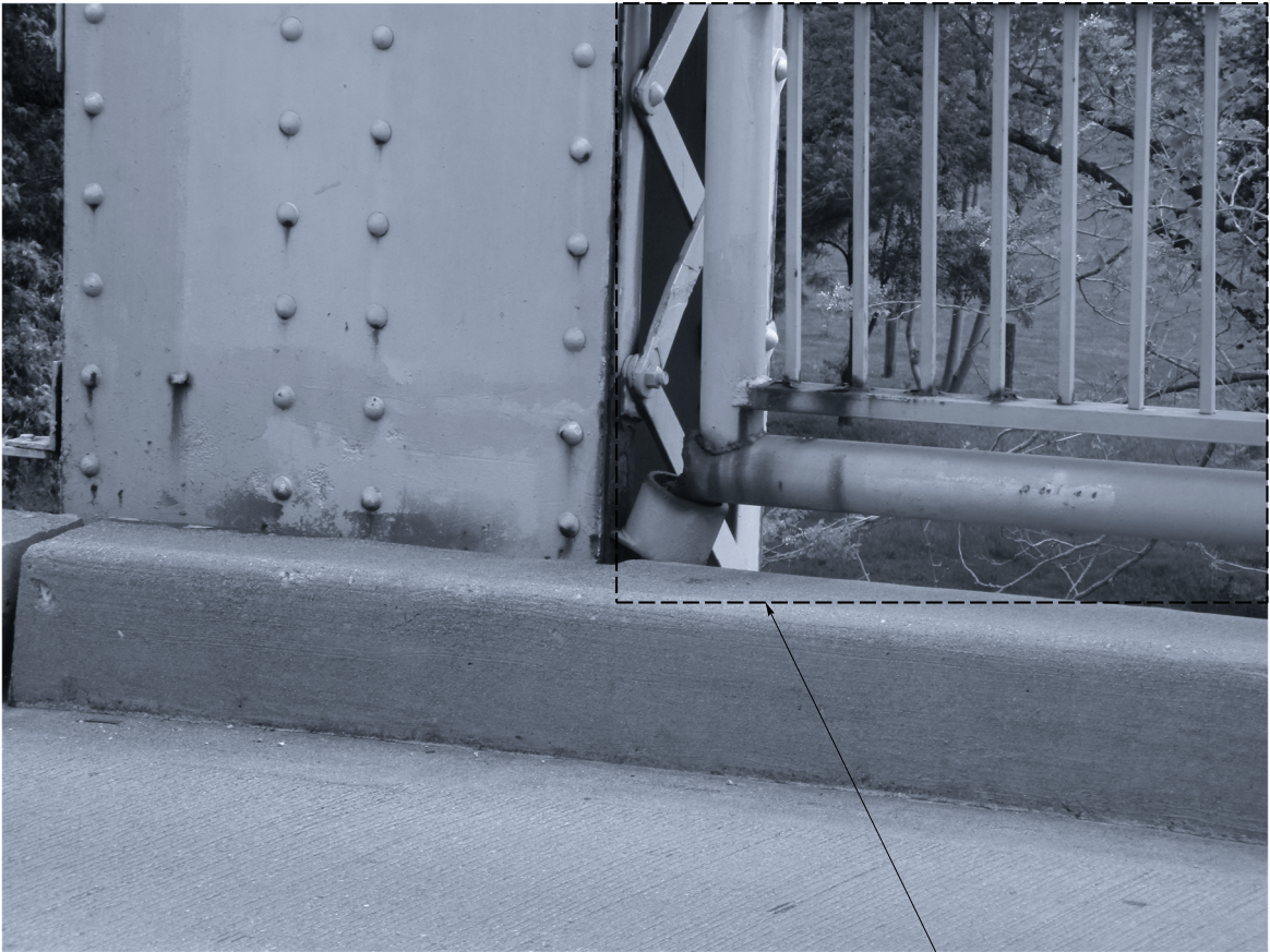
Repair Railing Connection
