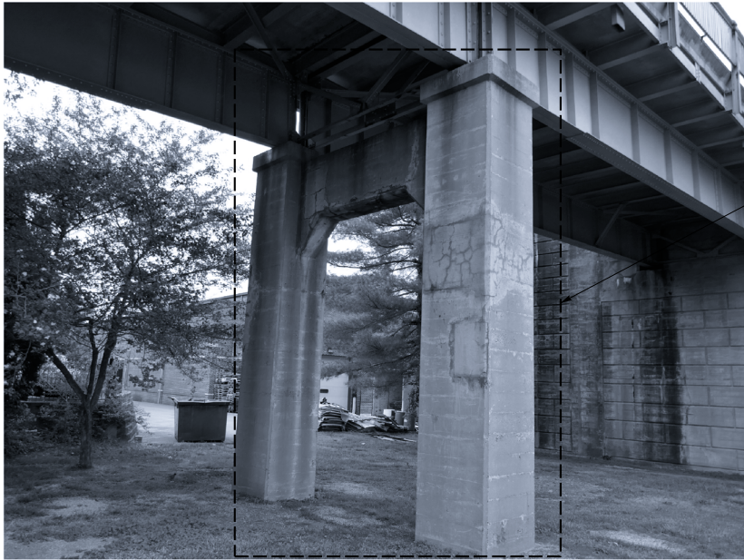
Concrete Patching and Coating of Substructure Units
