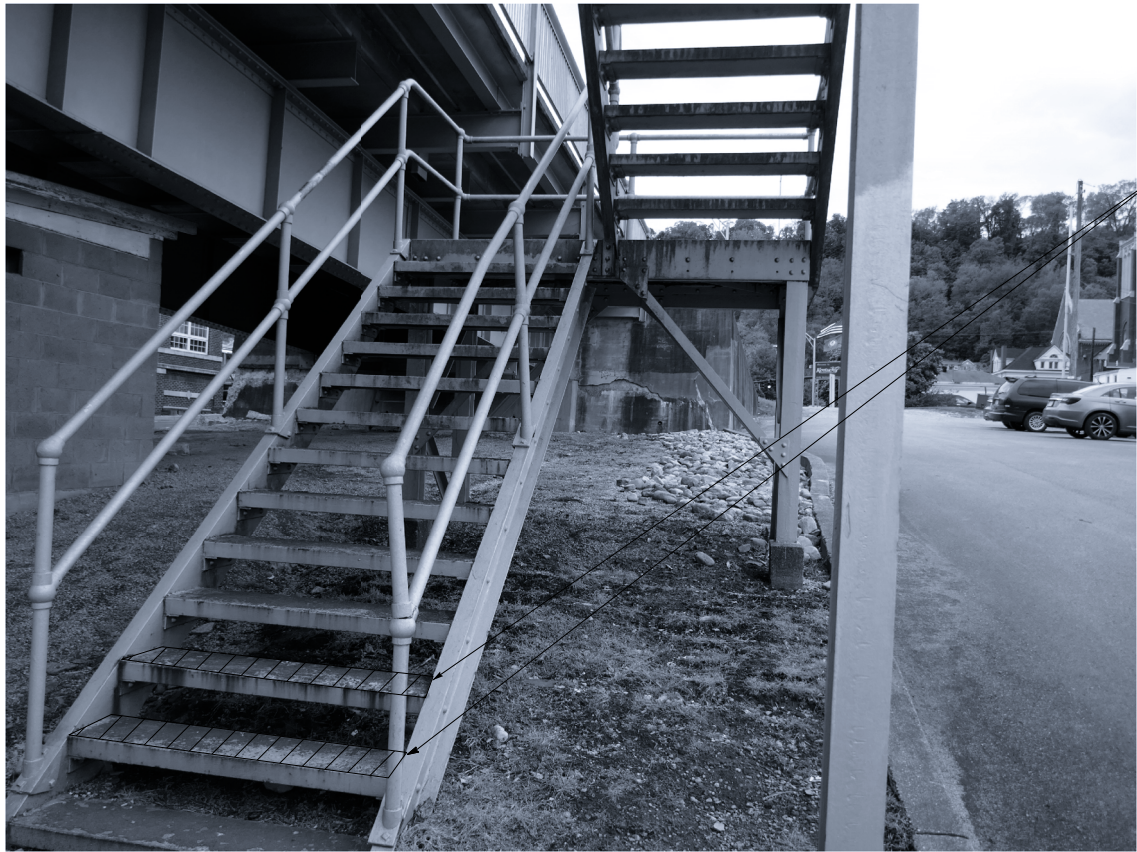
Repair Deteriorated Concrete Stair Treads
